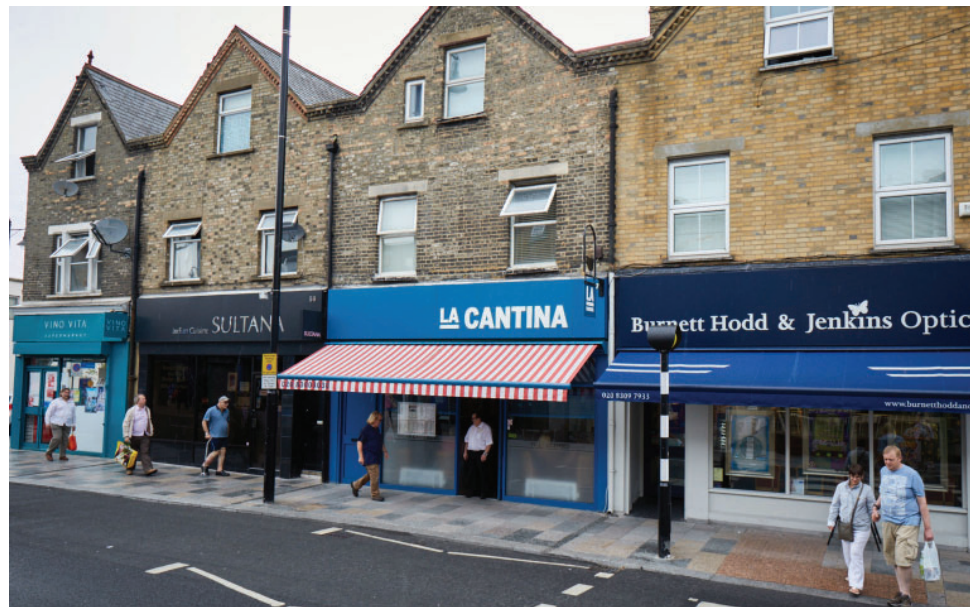
Unified shop fronts and high quality materials, Eastgate Street, Sidcup
