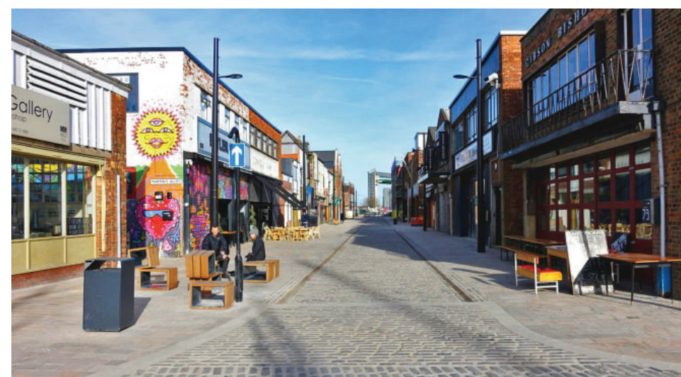
Improved shop fronts and shared surface, Humber Street, Hull
