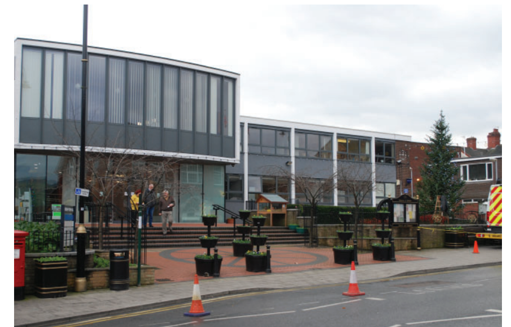
Before intervention; Space in front of the Town Hall
