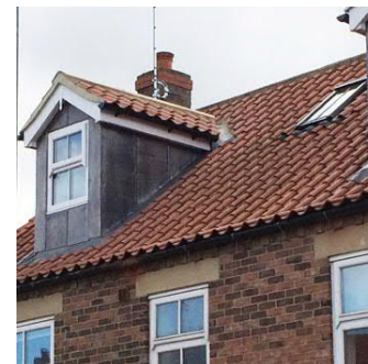
Gable end dormer window
