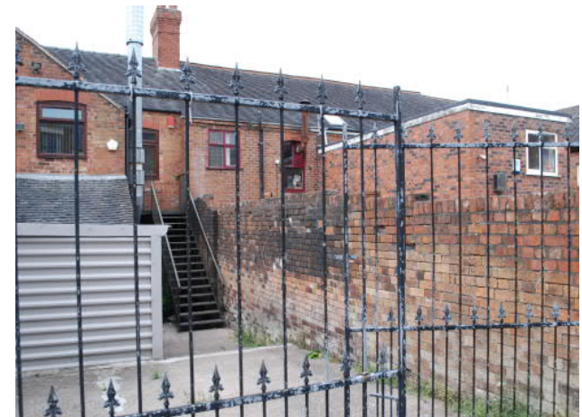
Rear access to residential upper floor, Biddulph High Street
