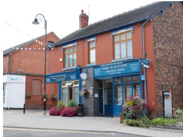
Commercial office units with retail facade treatment along ground floor providing coherence along street frontage, Biddulph High Street
