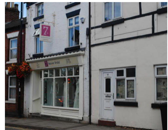
Boutique shop in residential area, Leek High Street
