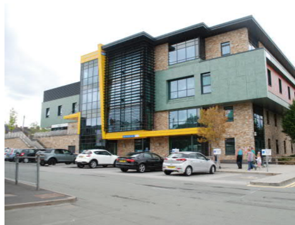
State of the art bespoke NHS building
