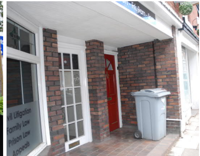
Office access on the ground floor and flats on the first floor
