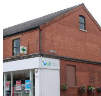
Side facing gable end
