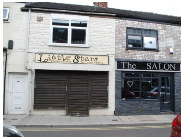
Discordant elevation styles within upper High Street
