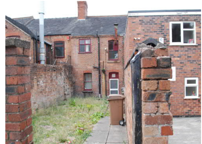
Rear of ground floor residential use along Biddulph High Street
