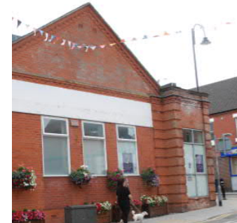
Gable end facing street
