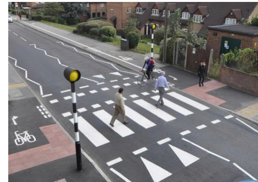
Raised pedestrian crossing
