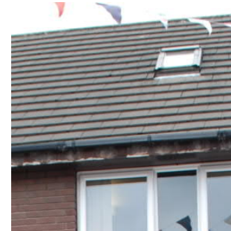
Roof light along front elevation
