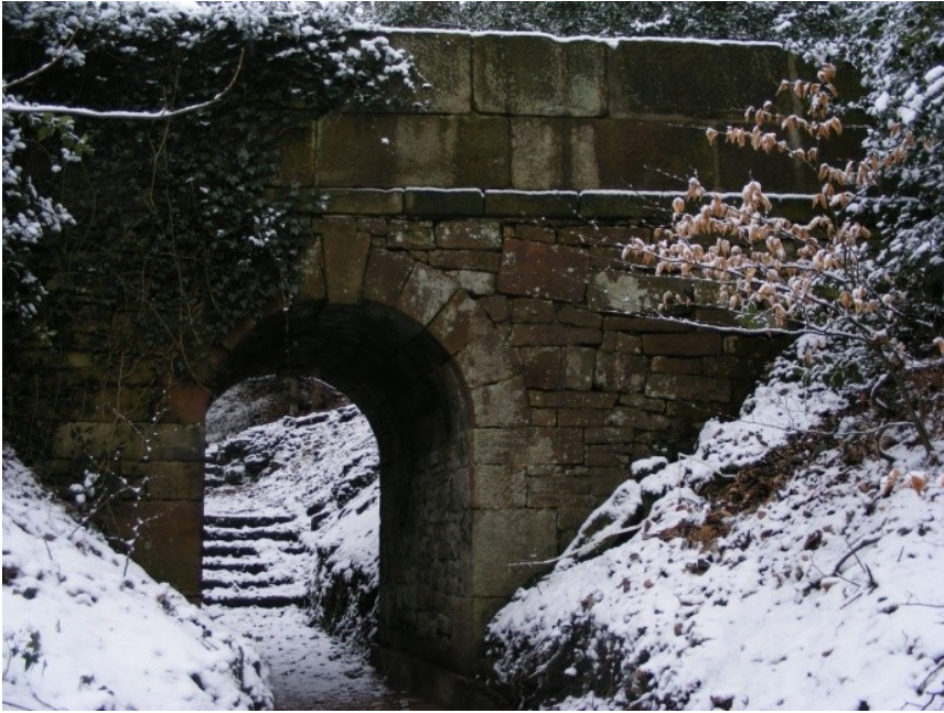
The existing bridge with footpath across the top
